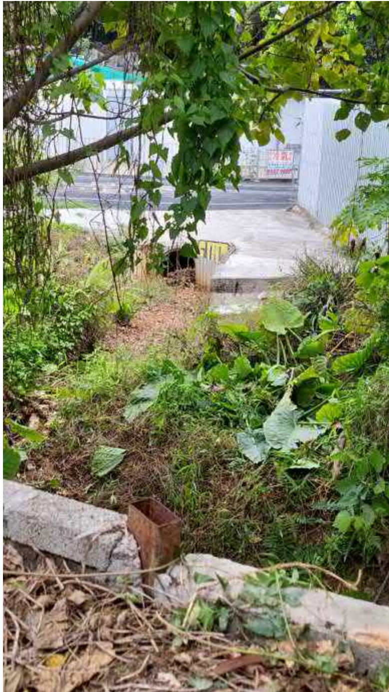
Photo 5 Existing open drain and connection to a 700mm diameter concrete pipe (Photo viewpoint is shown on the drainage plan)
